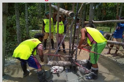
The borehole is part of a comprehensive WASH project for the host community in Bangladesh.
